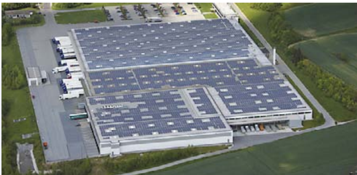
A photovoltaic installation of the DCM Solarfonds 1 on the roof of the ALDI logistics centre in Regenstauf, Bavaria.
